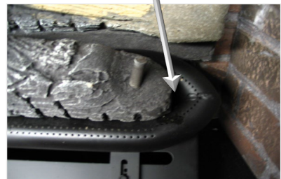
Push log "D" up against inside curve of burner.
