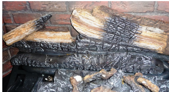
Push log "D" up against inside curve of burner.
